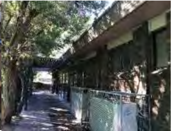
Fig 10 – Senior Citizens Centre External Lighting
