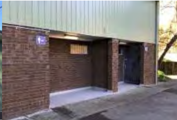
Fig 25 – Amenities building lighting
