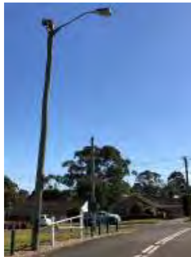
Fig 30 – John Wearn Reserve carpark lighting
