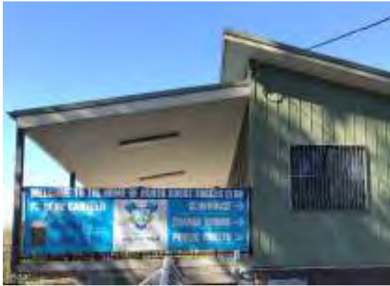
Fig 24 – Amenities building lighting
