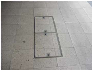
Paving infill lid in unit pavement
