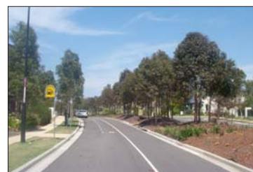
Asphalt roadway, Newington
