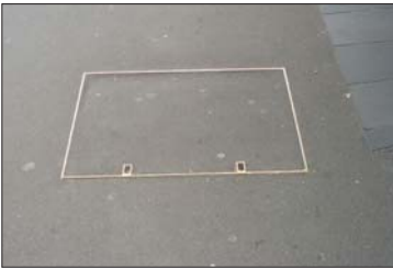
Paving infill lid in asphalt
