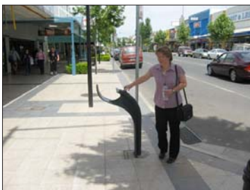
Exposed aggregate unit concrete pavement
