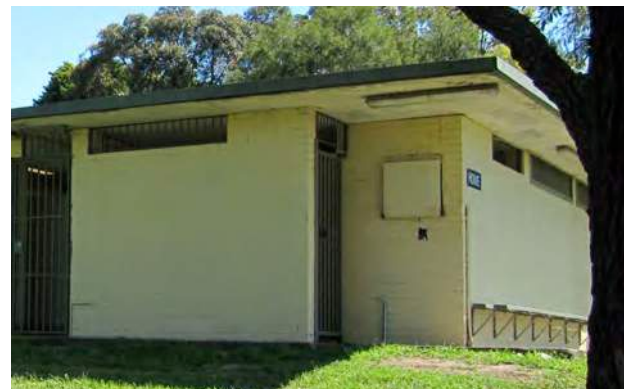
Security Lighting At Amenities Building - GKR
