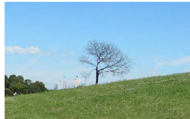
Dead tree: possibly landfill gas leak - GKR
