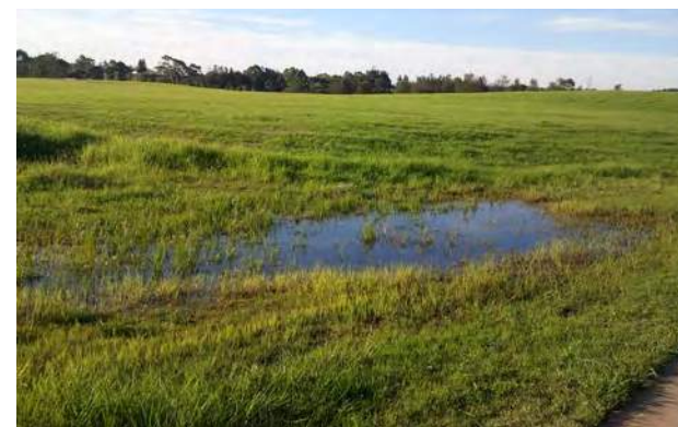
Ponding over landfill - GKR
