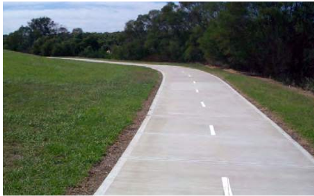
Parramatta Valley Cycleway - GKR
