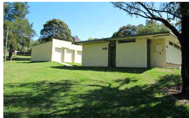
Amenities Building and Sports Storage - GKR
