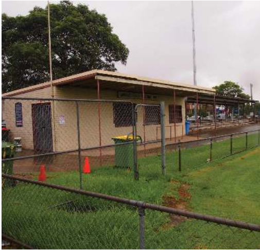
Former amenities building & covered seating
