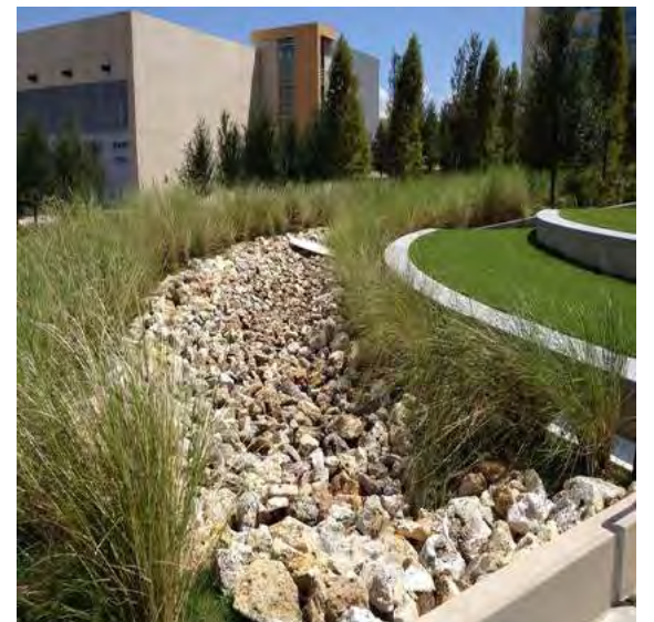
Infiltration beds with detention
