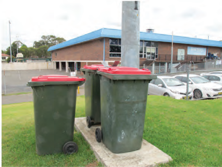
B6: 3 x sulo 240L bins. Concrete pad too small
