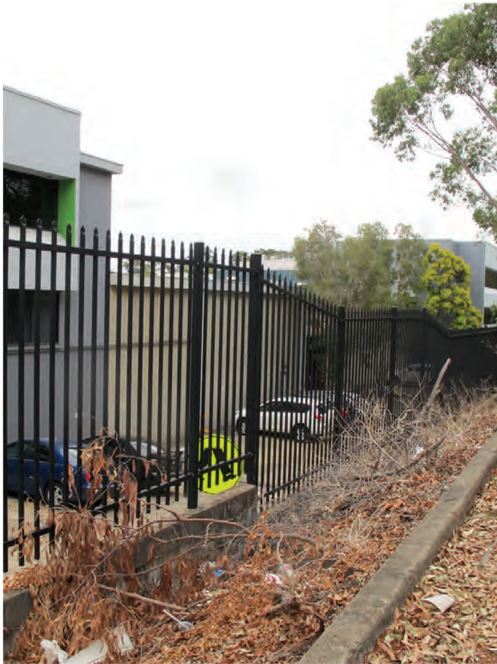
F6: High picket fence on high retaining wall. At southern end of site
