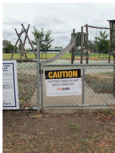
PE4: New fence. Childproof lock gate
