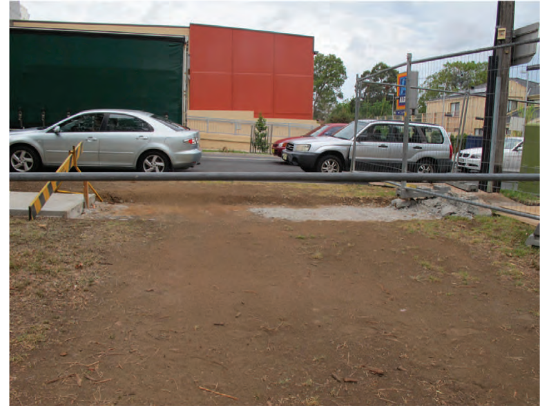
VC4: Under construction . Metal beam ga
