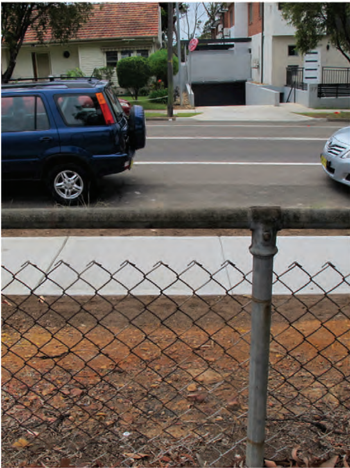
F3: Mesh separating from top bar
