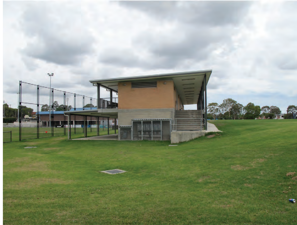
D1: New stormwater drains
