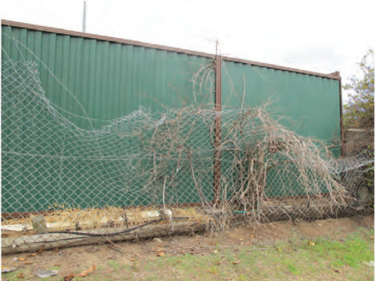
Bowling Club: Fences near ST2. Perimeter F1 damaged
