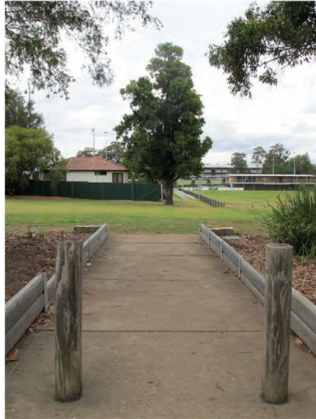
PE 2 : Concrete path with timber bollards
