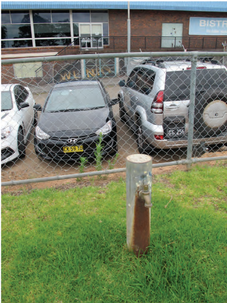
WP1: Brass garden tap on metal and concrete post. No handle
