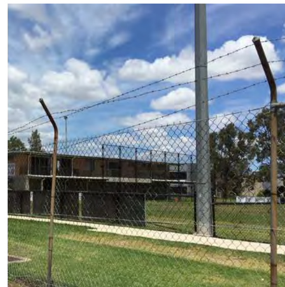
Existing club house
