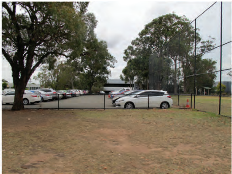
F4: New wire mesh fence with high section
