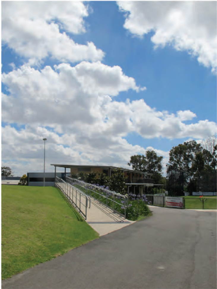
A1: Accessible ramp
