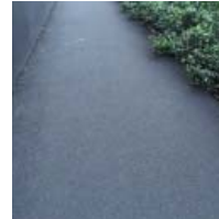
Railway corridor Material: asphalt concrete of AC10 and AC5 (wearing course) Colour: natural
