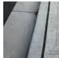
Kerb & gutter Material: concrete
