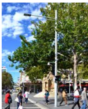
Large Multi Functional Pole (10m)
