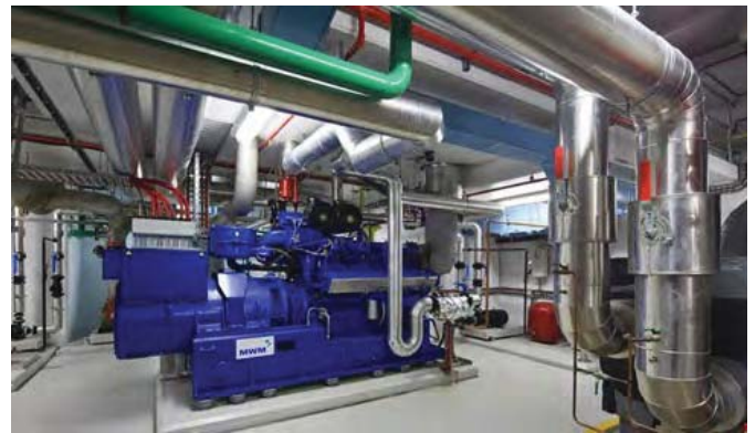
Tri generation energy plant
