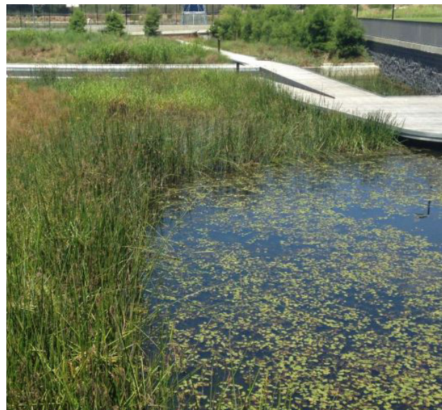
Figure 4.23 Stormwater treatment system at Blacktown Showground
