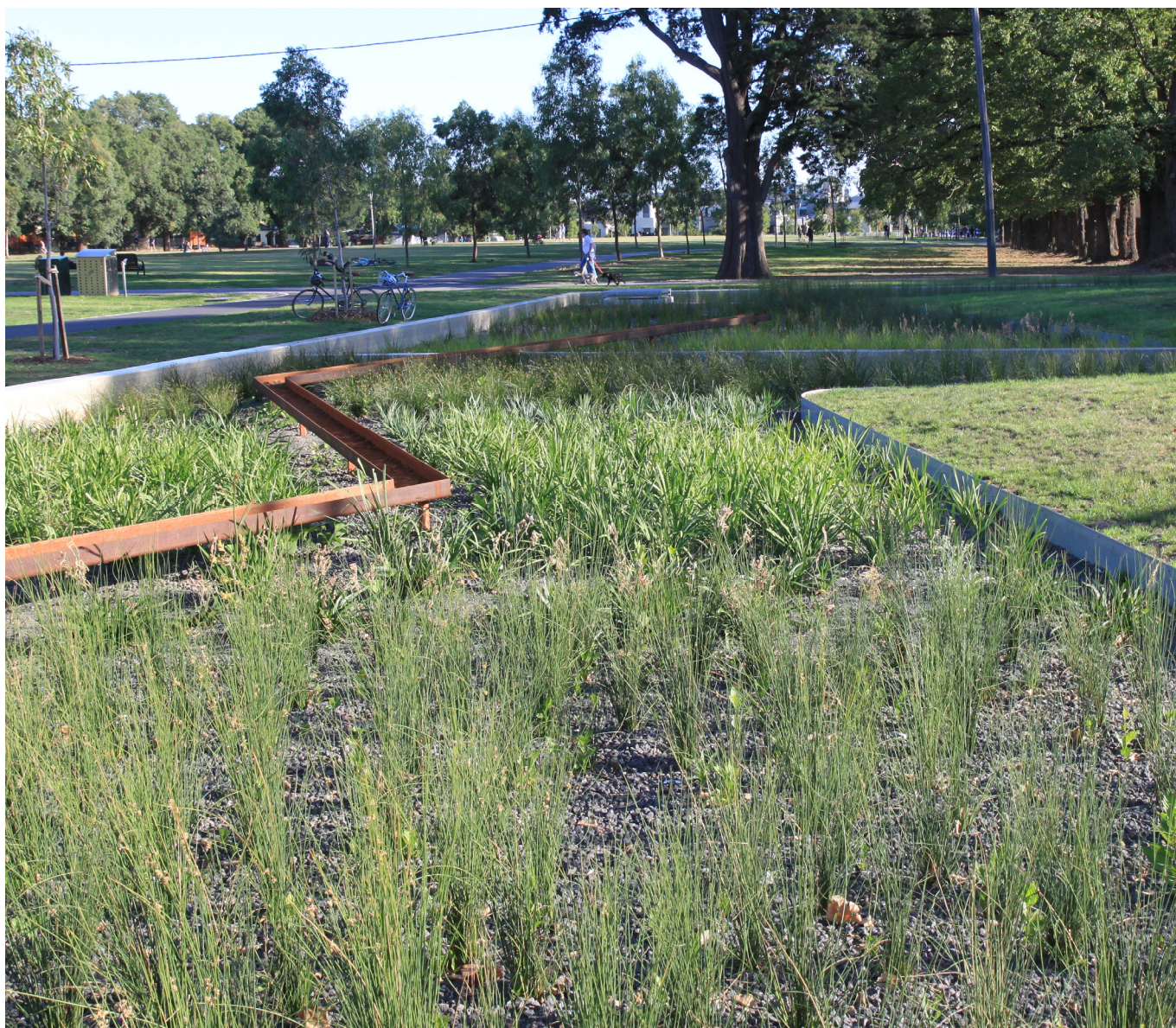
Figure 4.16 Biofiltration at Edinburgh Gardens, Melbourne
