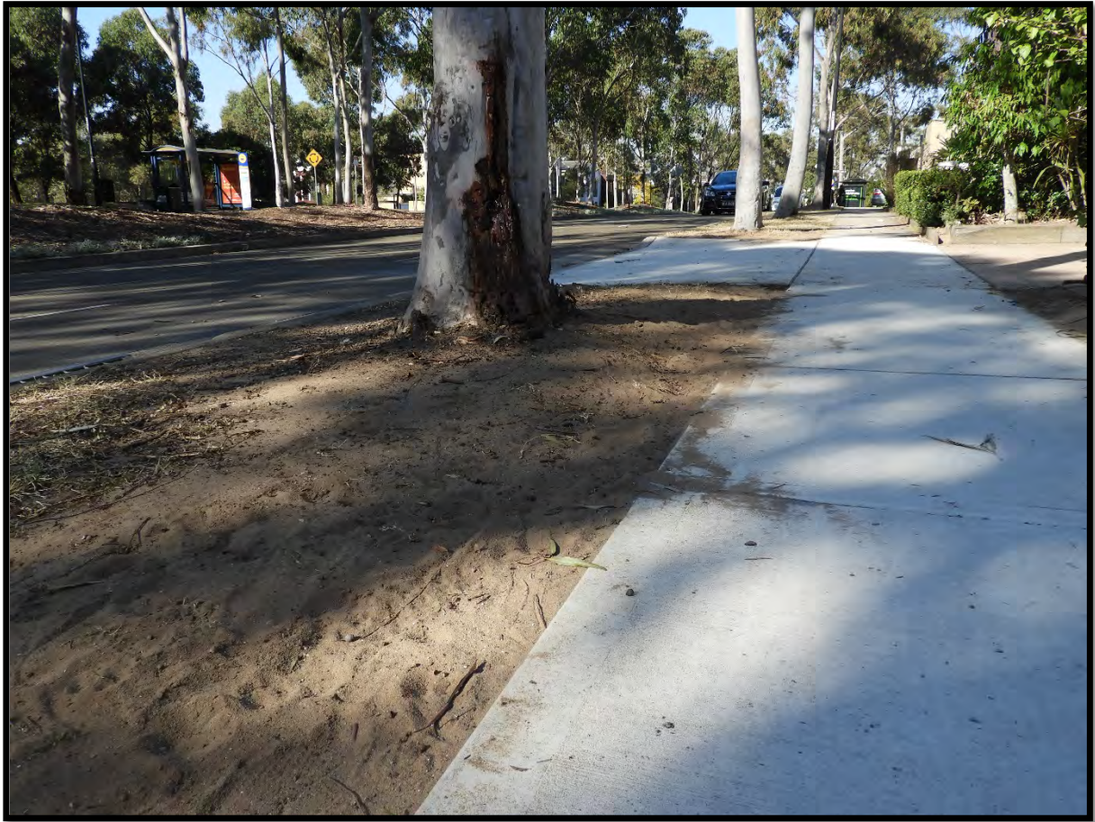
An example of both tree being planted too shallow and newly installed footpath. The construction of the footpath appears to only have regular expansion joints and no Tripstop.
