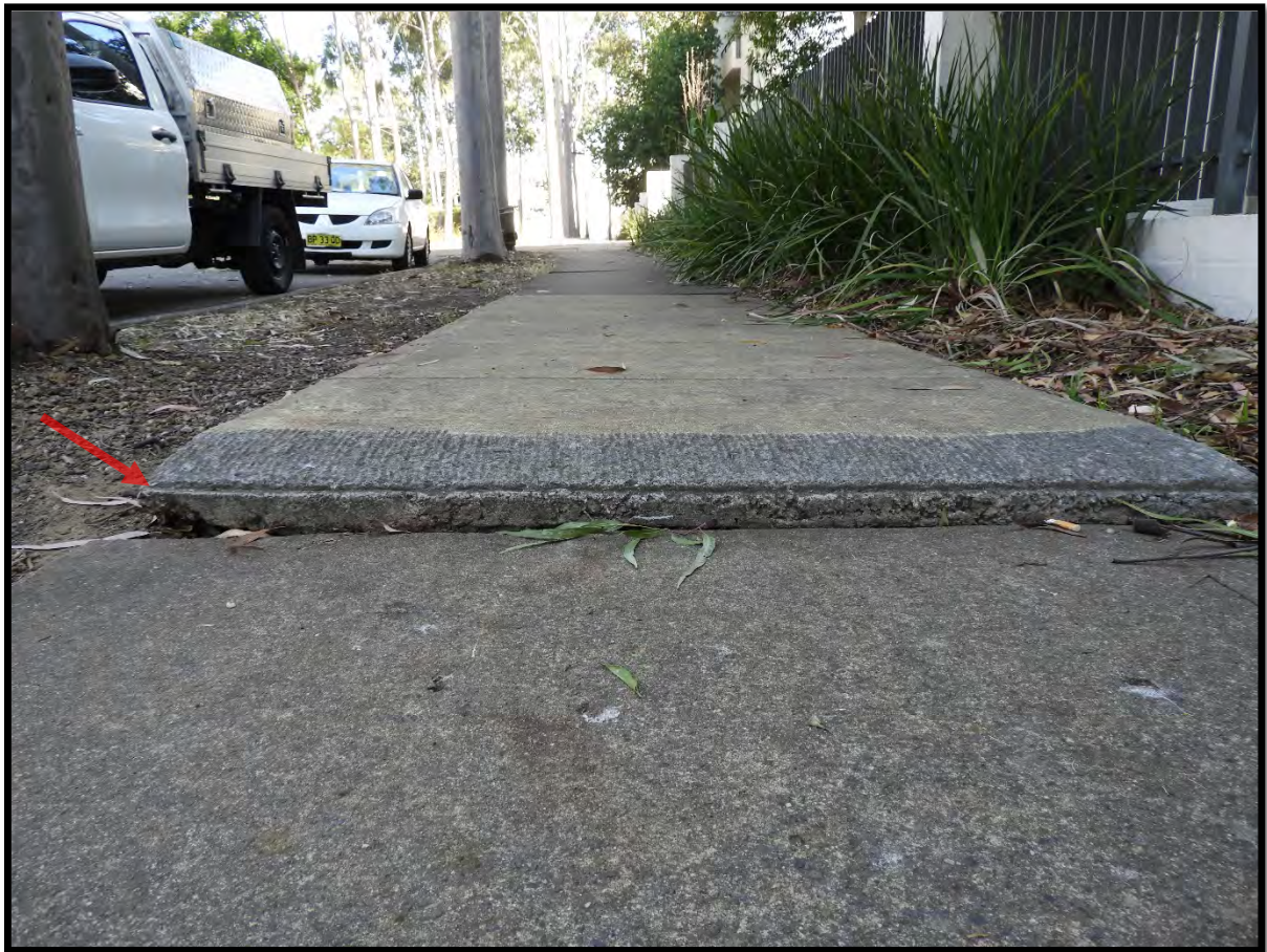
An example of significant foot path displacement. This is also an example of a Priority 2 Tree as repairs to the footpath will likely cause significant damage to the tree's structural root system.
