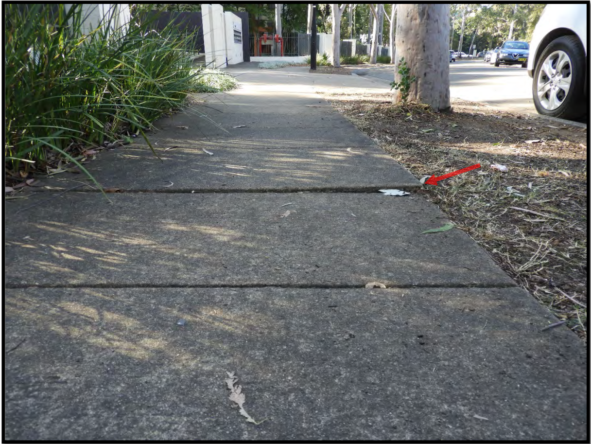
An example of minor footpath displacement. This is also an example of a Priority 4 Tree.
