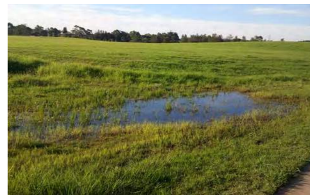
Ponding over landfill - GGRP
