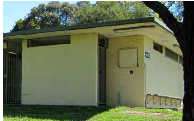
Security Lighting At Amenities Building - GKRP
