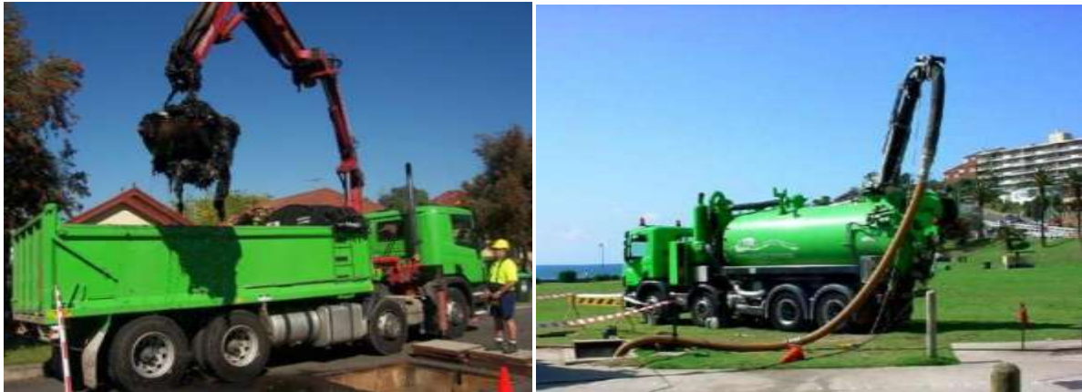
Figure 63. CDS GPTs can be cleaned using a grab arm or a suction cleaner.
