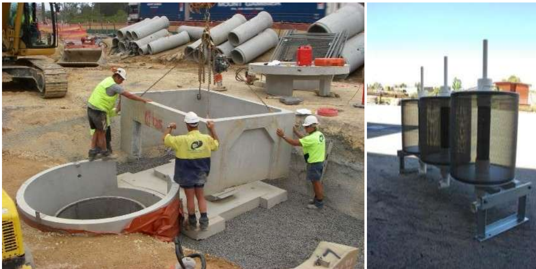
Figure 61. Precast diversion units can be installed almost anywhere; the filternator sits inside the unit and screens bulk solids from stormwater.
