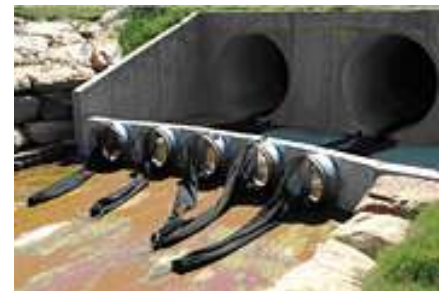
Figure 64. Retrofit Pratten Traps.
