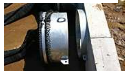
Figure 65. Detachable traps are easy to maintain, but secure.
