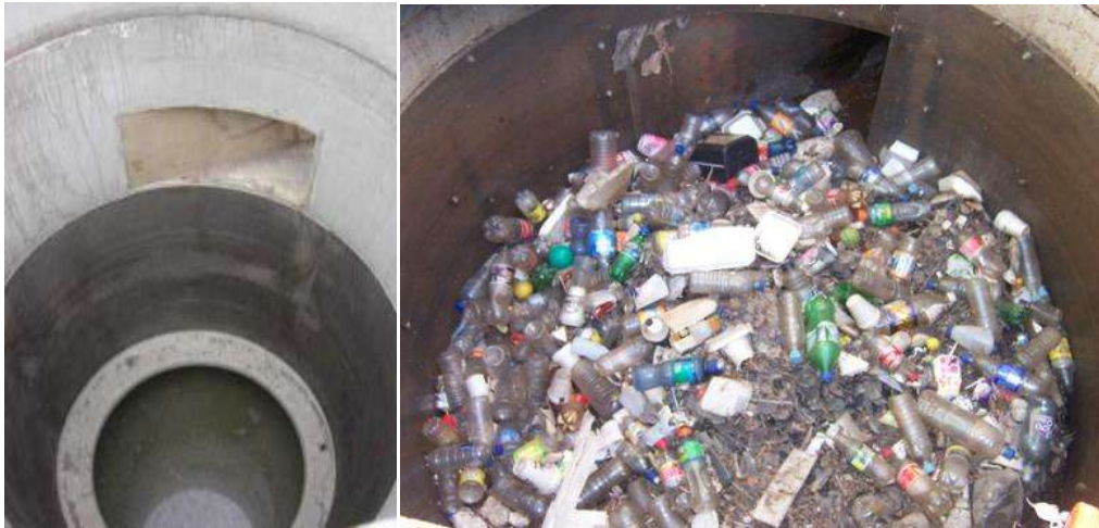
Figure 60. Rocla's CDS 0708: empty, and full of gross pollutants.
