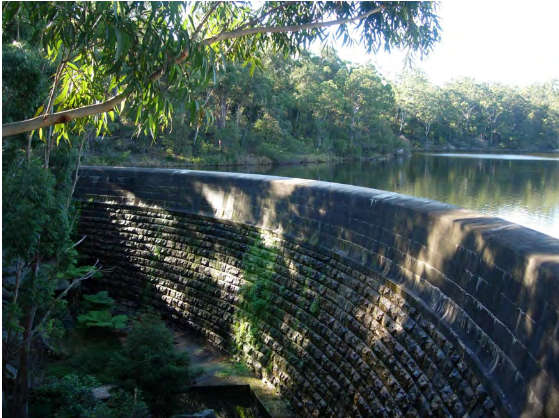
Photo: Lake Parramatta Dam Wall
