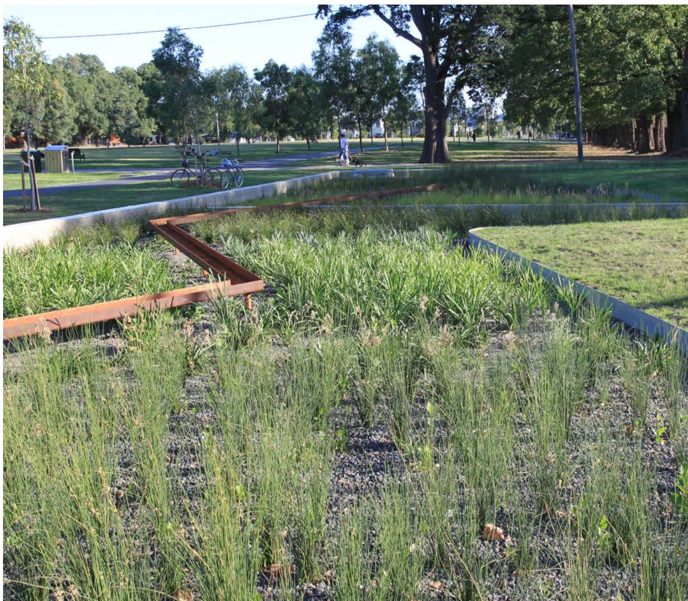
Figure 4.33 Biofiltration at Edinburgh Gardens, Melbourne
