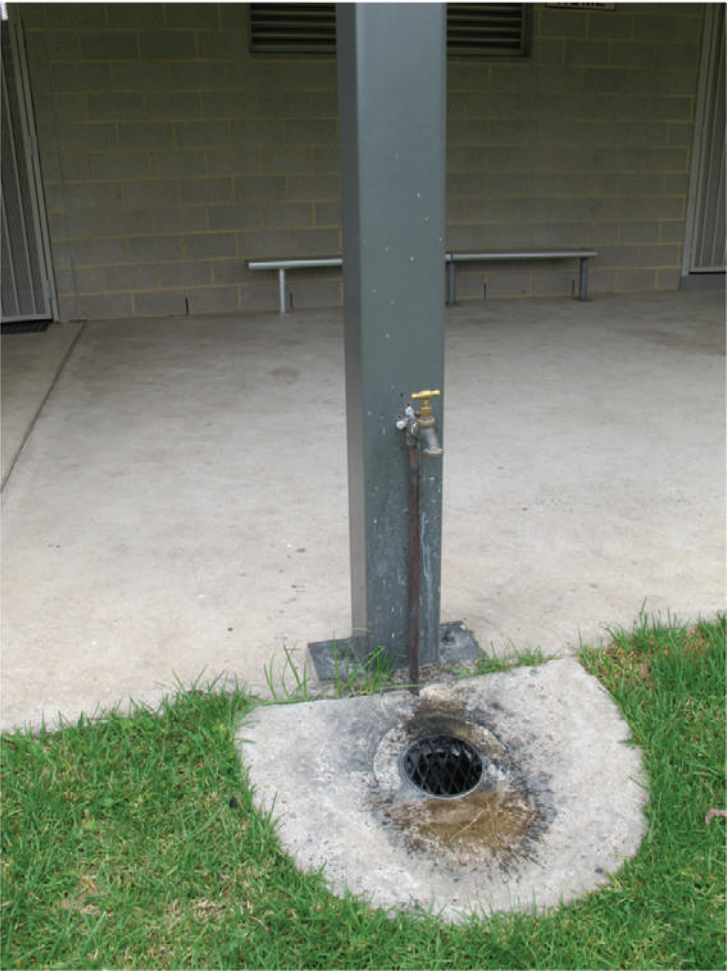
WP9: Brass garden tap on steel column. Drain underneath
