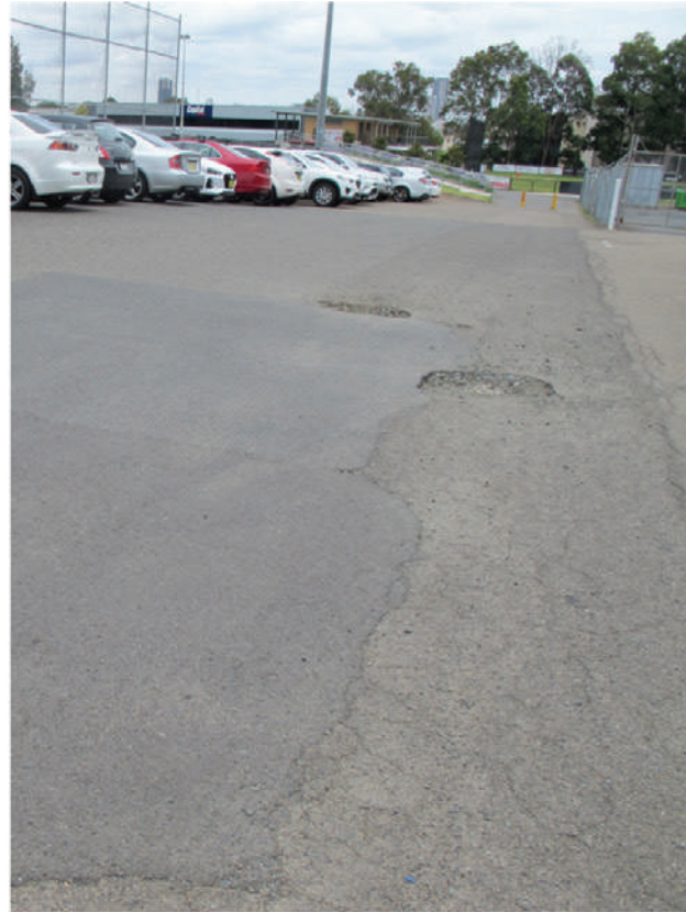
CP1: Patched bitumen with large potholes
