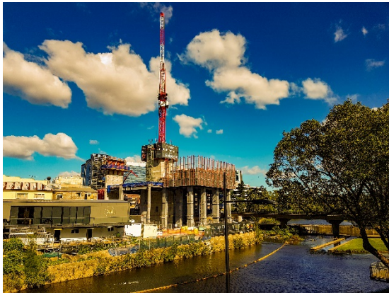
Figure 29 – New 46 storey mixed use tower under construction behind heritage listed shop buildings on Church Street
