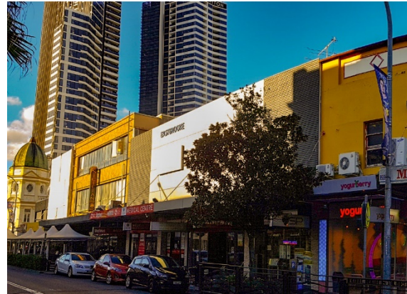
Figure 26 – Existing commercial and shop buildings on Church Street (looking north towards Phillip Street)
