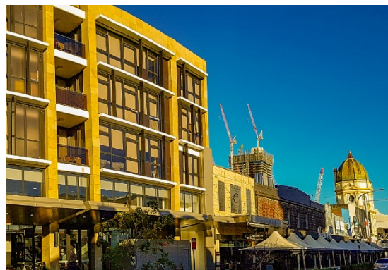
Figure 32 – View looking south along Church Street (from the river)
