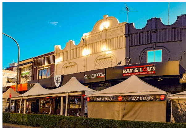
Figure 28 – Heritage listed shop buildings on Church Street (showing outdoor dining)
