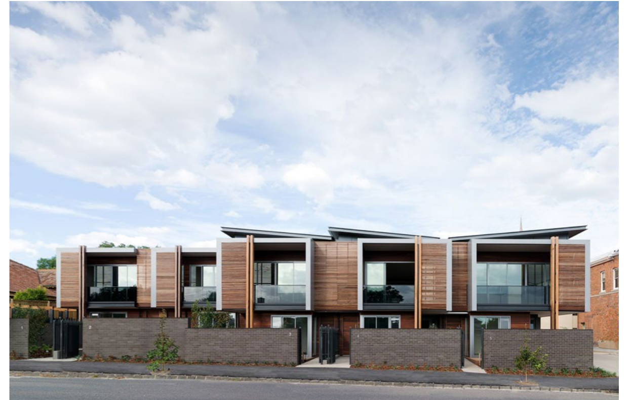
Kew Townhouses - SJB Architects
