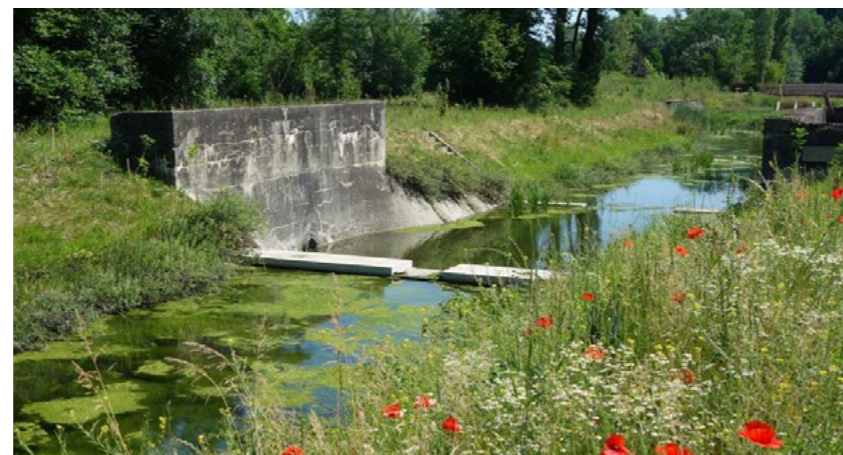
River Aire Regeneration, Switzerland
