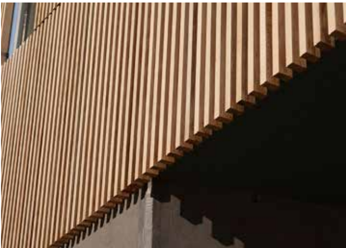
06 Timber battens on aluminum framing
