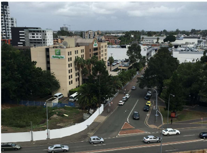
Figure 3 – Site seen from intersection of Anderson St and Parkes St (looking south)
