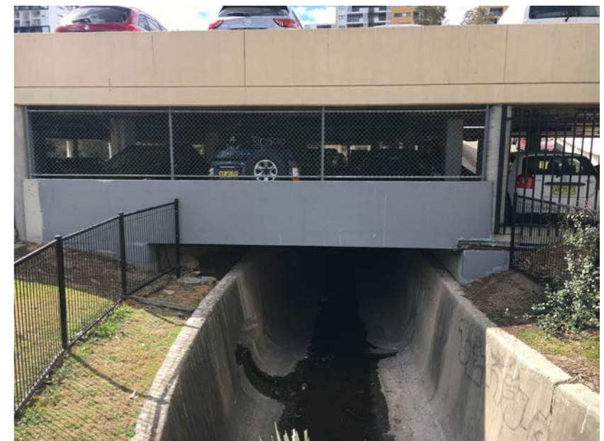
6. Clay Cliff Creek at Anderson St
