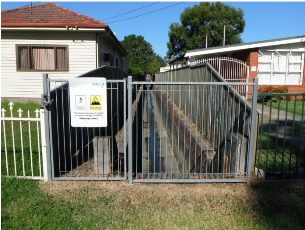
Figure 21. In many cases there is little room between the channel and surrounding development (UNNAMED 8 GUILDFORD RD)
