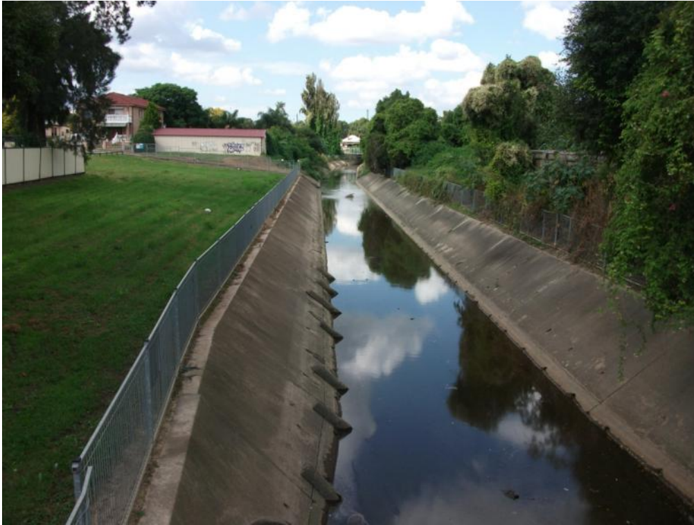
Figure 20. Larger channels in the lower catchment include reach A'BECKETTS 1, with an open space corridor
