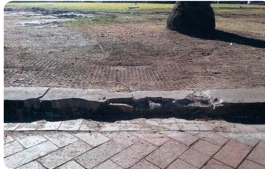
Damage to the sandstone edging due to vehicles driving over the edging.
