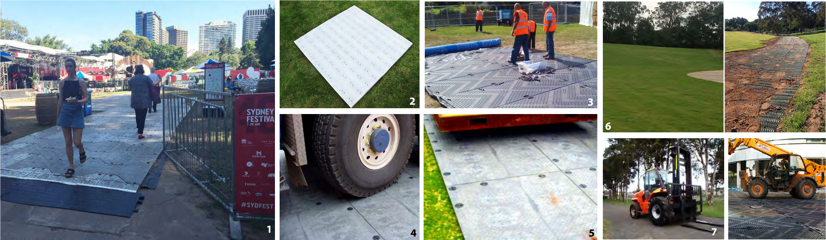
Examples of ground protection during events: Ground protection used at Hyde Park, Sydney (1) Terra plas (2), Zigma (3) Terratrak plus (4 and 5) and. Grass Reinforcement Mesh before and after installation at Parramatta Park Trust, Crescent Amphitheatre (6) Manitou Forklifts with all terrain tire required to be used on turf areas in Hyde Park (7)
