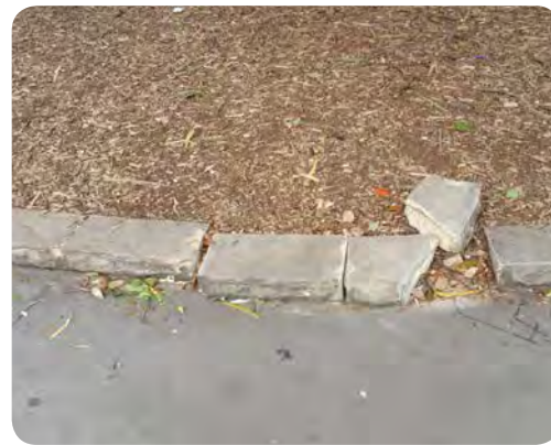
Much of the sandstone edging is damaged from vehicles and the nature of the soft material
