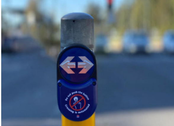
Figure 1: A semi-permanent plastic cover installed over the 'push' button
