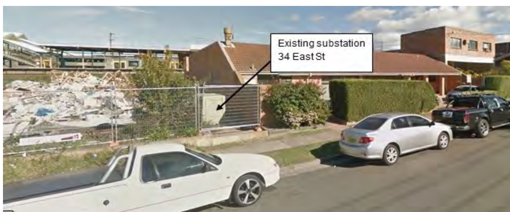
Figure 4.3.7.2.4 Existing padmount substation at 38 East Street, Granville
