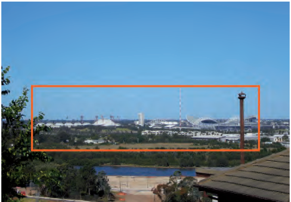
Figure A2.2.11 Looking South towards the Homebush Olympic site, Coffey Street, Ermington
