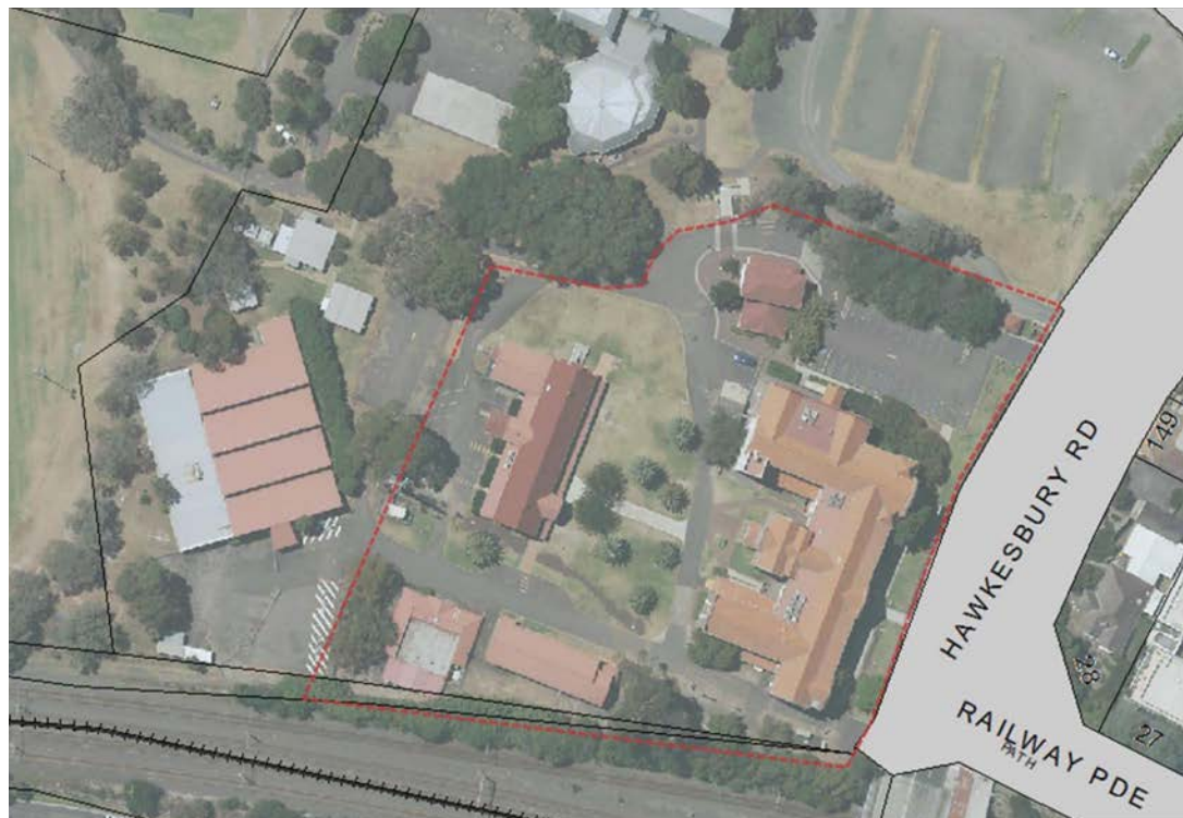
Figure 4.3.4.1.5 Aerial View Demonstrating the Curtilage of the Buildings of Heritage Significance
