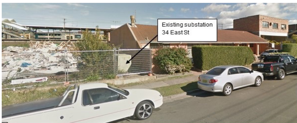
Figure 4.3.7.2.4 Existing padmount substation at 38 East Street, Granville
