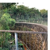
A concrete rim adding 3.3m to the dam height was built in 1898.
