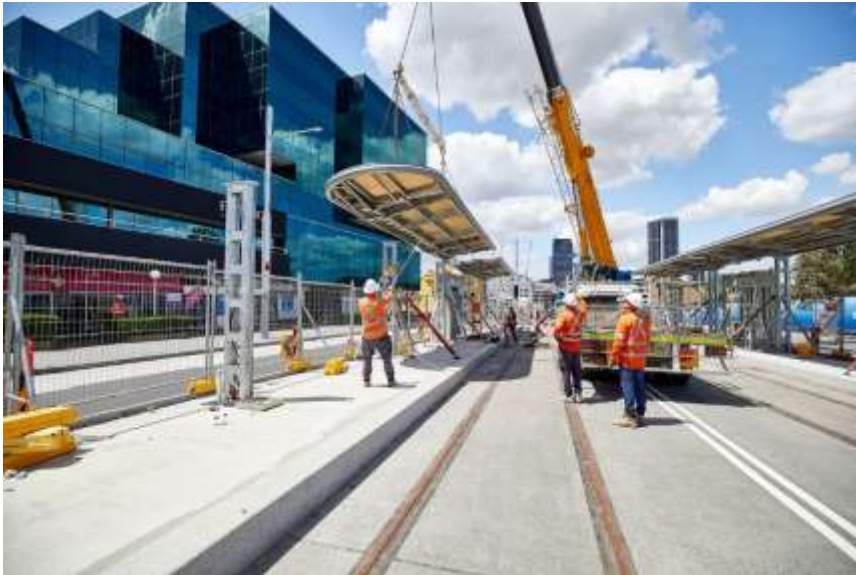
Canopy installation at the Fennell Street light rail stop.
