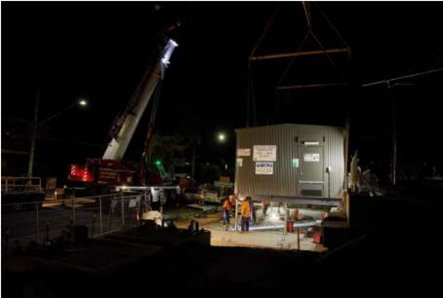
The pre-fabricated Telopea substation building was craned into place.
