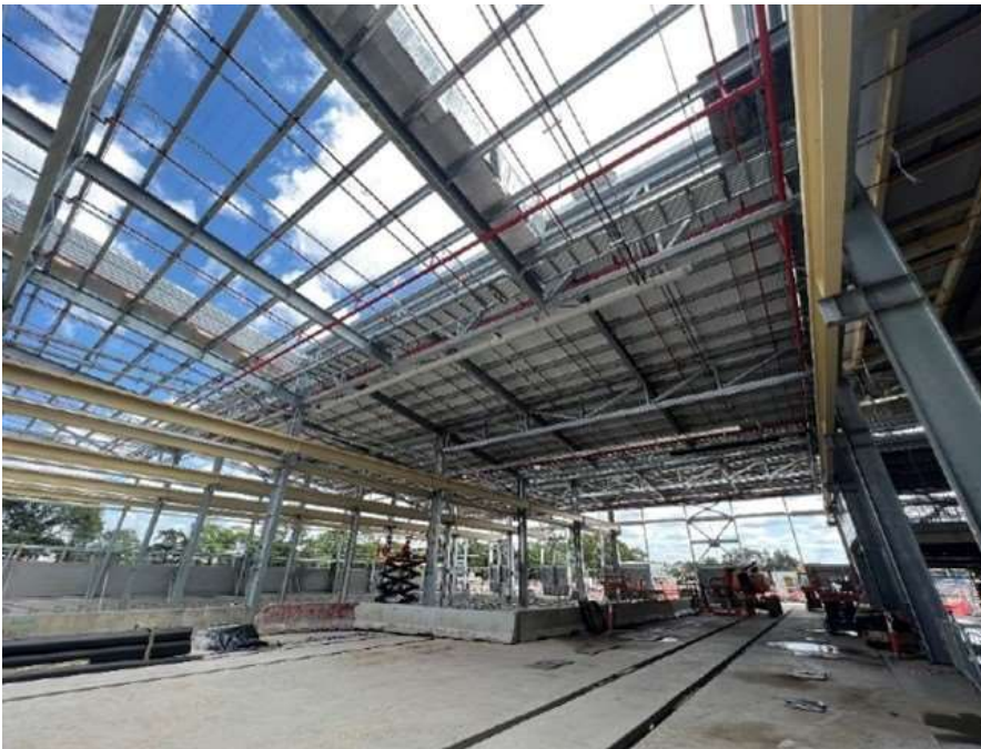
Roof panel installation on the maintenance workshop.
