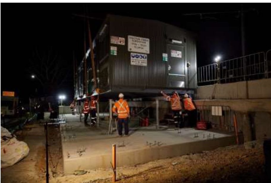
The building has been placed on a concrete slab.
