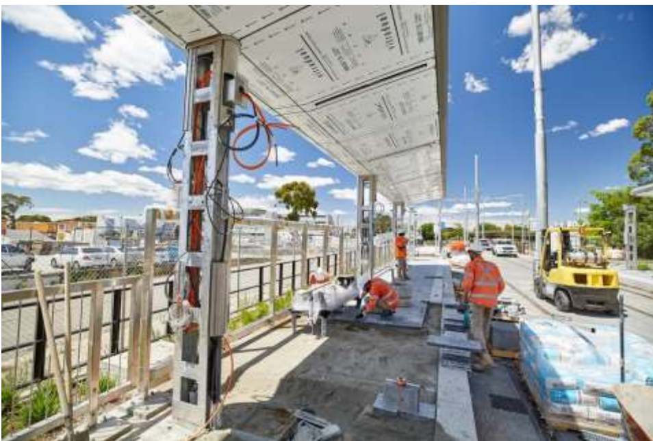
Paving is underway at the Rosehill Gardens light rail stop.
