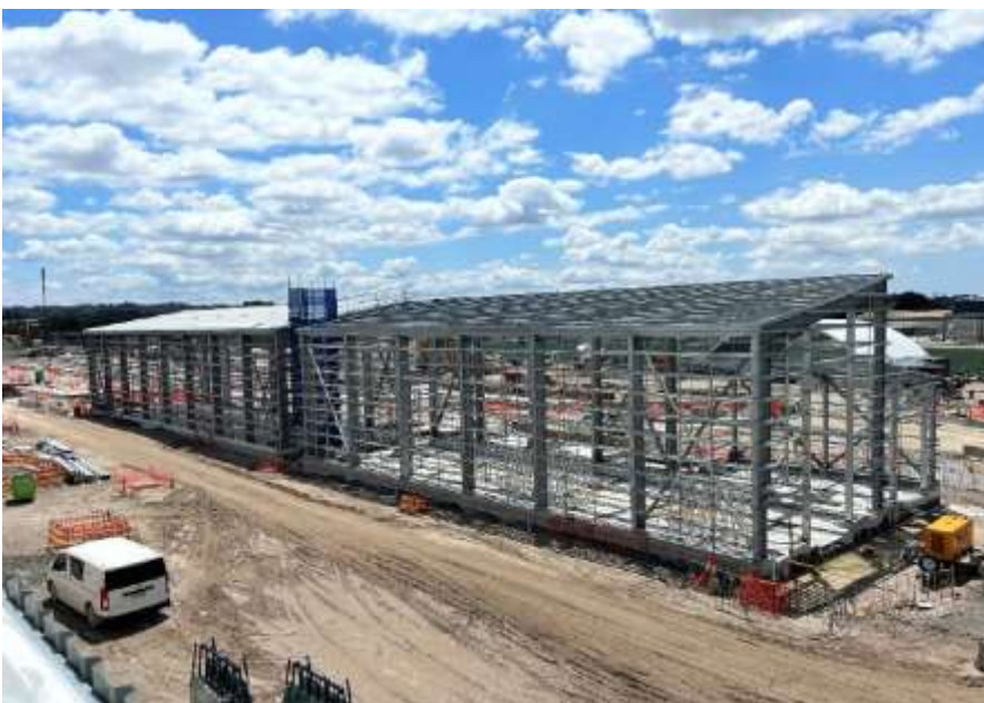
The light rail wash facility is taking shape.
