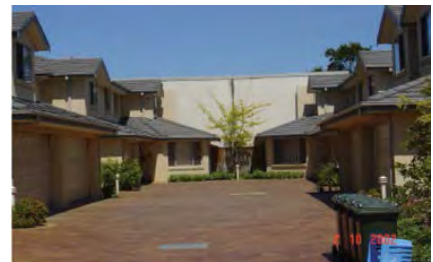
Figure 4: Poor residential/industrial interface
