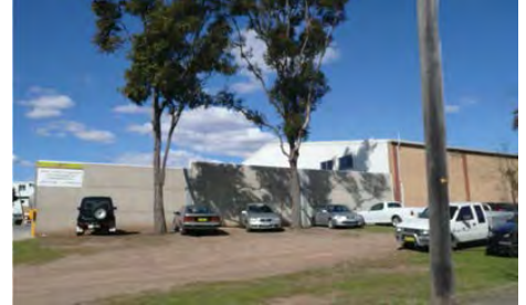
Figure 2: Poor example of blank wall treatment
