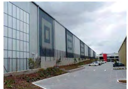
Figure 3: Good example of blank wall treatment
