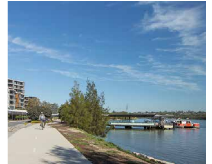
Ferry Terminal, Wentworth Point
