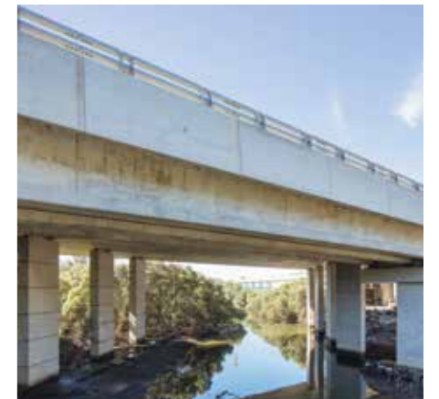
M4 Westconnex Overpass
