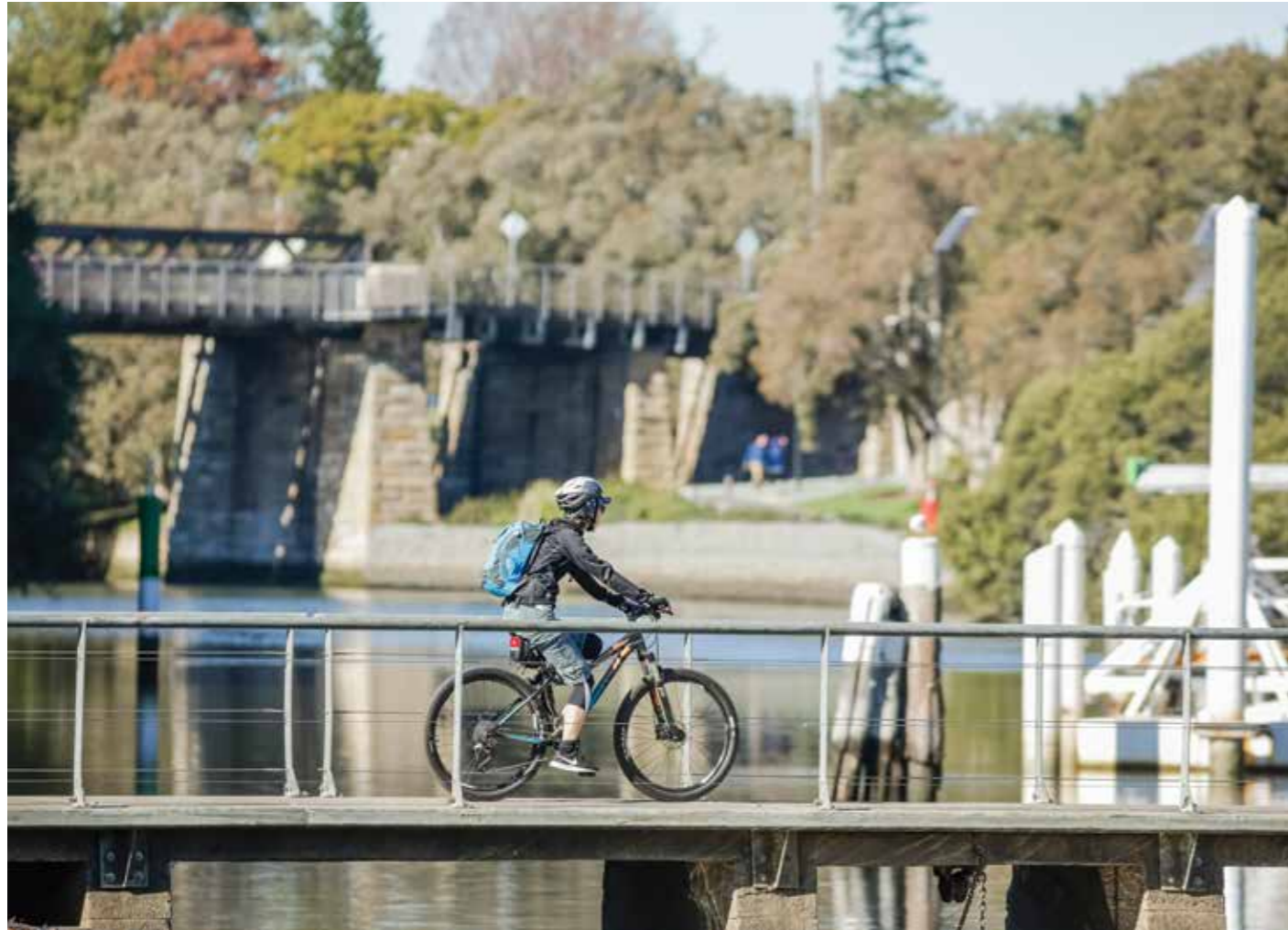
Charles Street Weir
