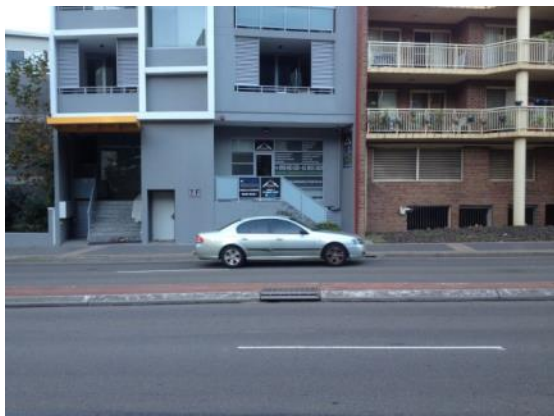
Figure 4: Fire Exit and Ground Level Example 1
