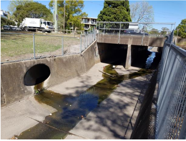
Figure 1-37 Circular and box culverts at Finlaysons Creek looking upstream
