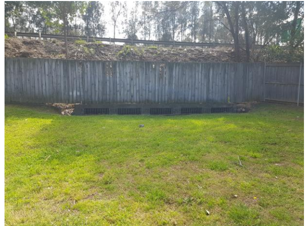
Figure 1-35 Brickfield Basin culvert total grate openings
