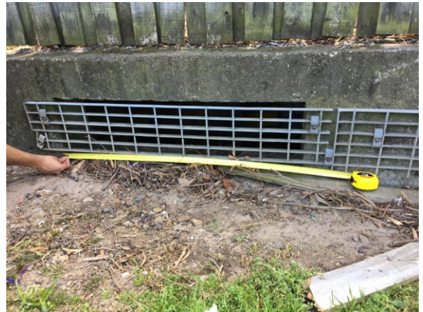
Figure 1-34 Brickfield Basin culvert grate open dimension inspection
