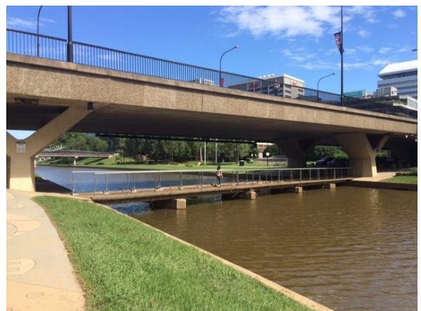
Figure 1-6 Footbridge under Wilde Avenue Bridge. The piers of both the footbridge and the road bridge need to be considered for modelling
