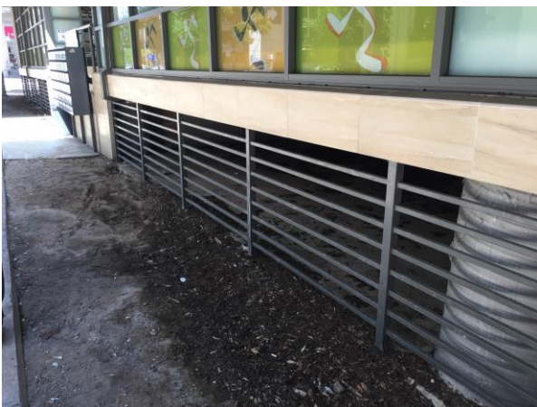
Figure 1-15 Culvert and grate at the intersection of Cowper and Parkes St
