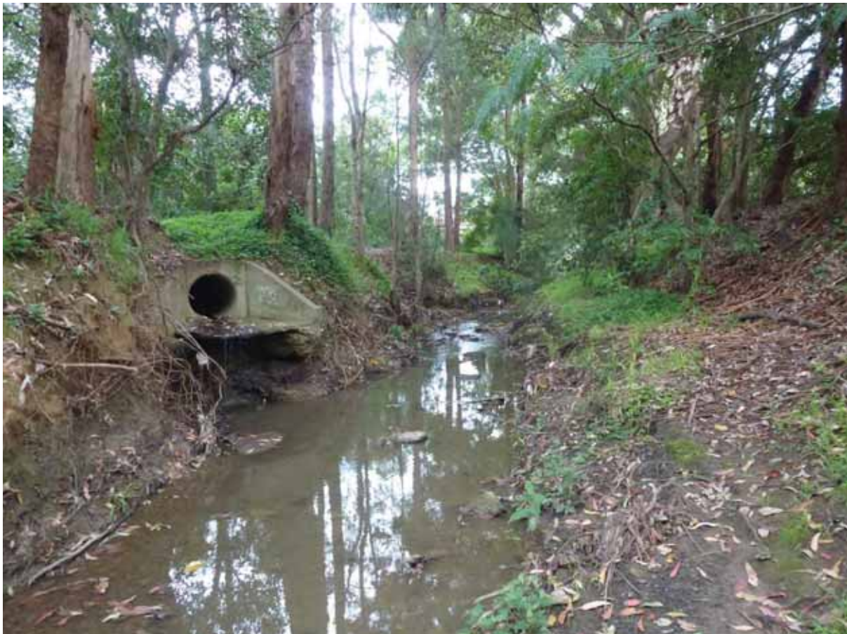
Figure 33 Higher rainfall intensities and increases in peak flows will lead to more erosion such as this scouring around a pipe outlet at David Hamilton Reserve
