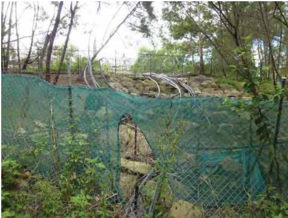
Figure 8 The Brickworks detention pond has numerous PVC pipes assisting with dewatering following a recent storm
