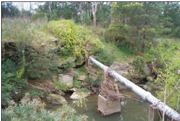
Plate 5 Site of Sewer Aqueduct
