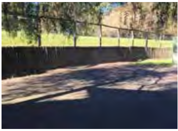
Treated pine log retaining wall
