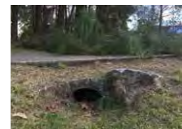
Turf swale with drainage under path
