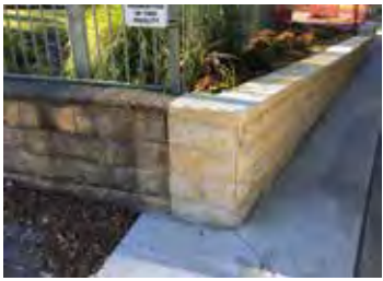
Sandstone capped retaining wall
