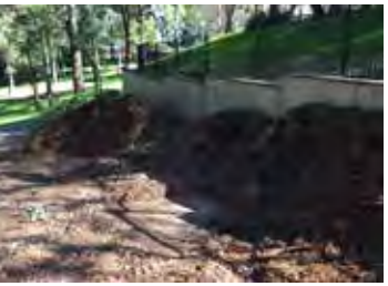
Concrete block retaining wall
