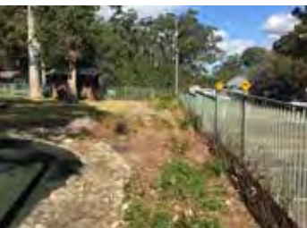
Informal drainage line with rock finish
