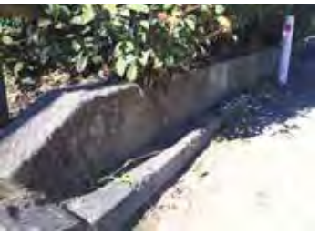
Sandstone block retaining wall
