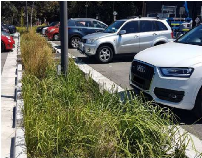
Figure 8.2.6.8.6.2 – Stormwater Swales (Source: Sydney Water – 'Water Sensitive Urban Design' SW277 03/18)
