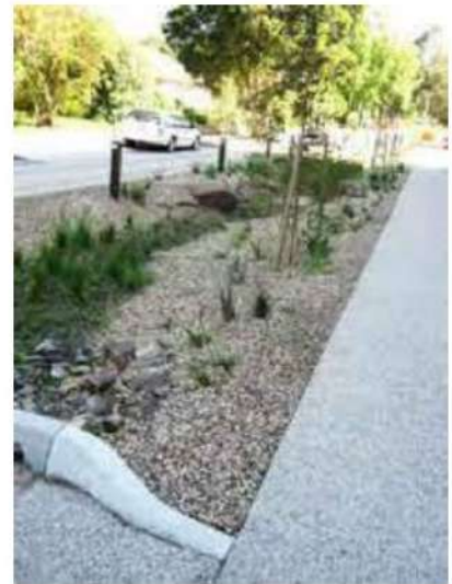
Figure 8.2.6.8.6.2 – Stormwater Swales (Source: Sydney Water – 'Water Sensitive Urban Design' SW277 03/18)
