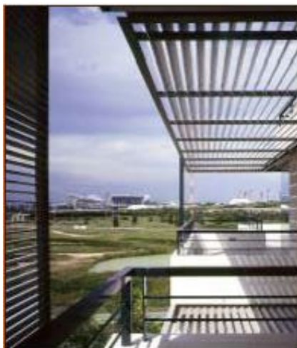
Figure 8.2.8.1.10.1 – Provide residents with means to adjust the quantity of daylight (Source: Residential Flat Design Code )
