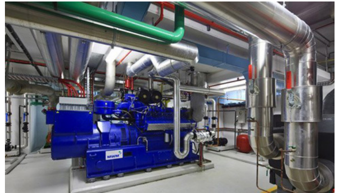
Tri generation energy plant
