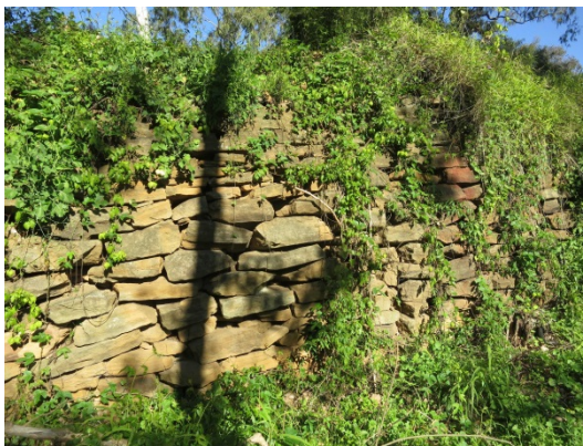
E-15 Part of one of the sandstone retaining walls constructed along Darling Mills Creek embankment (left) and evidence of a post hole cut into the sandstone of Darling Mills Creek (right) Source: TKD Architects 2015.
