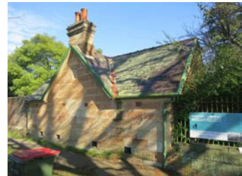
The Gate Lodge (N07), constructed c1860.
