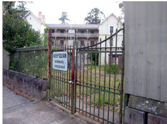
74 The sandstone and cast iron palisade fence with later gates and other openings. Source: TKD Architects, 2015.
