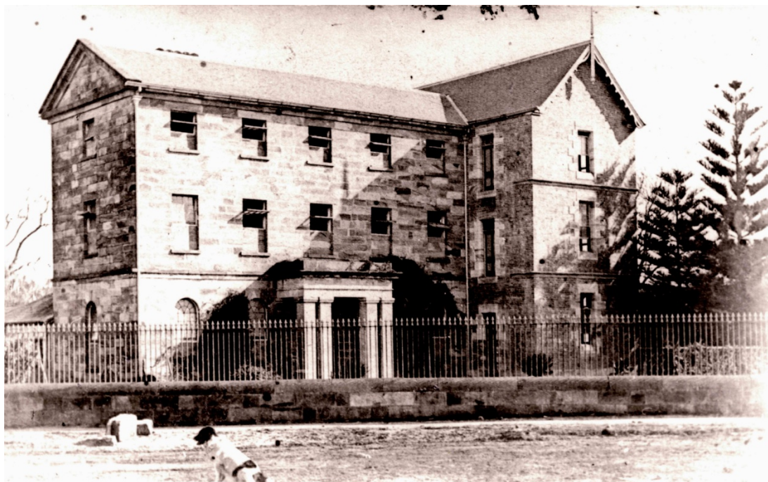
14 c1870 view of the main building after completion of Munro's three-storey North Wing addition. Source: SAG 5/9304B.
