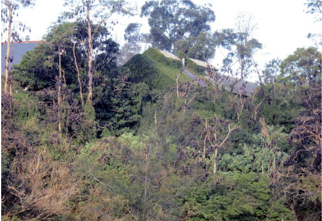
68 Glimpses of the roof of the Southwest Range and Laundry Building from Wistaria Gardens. Source: TKD Architects, 2015.
