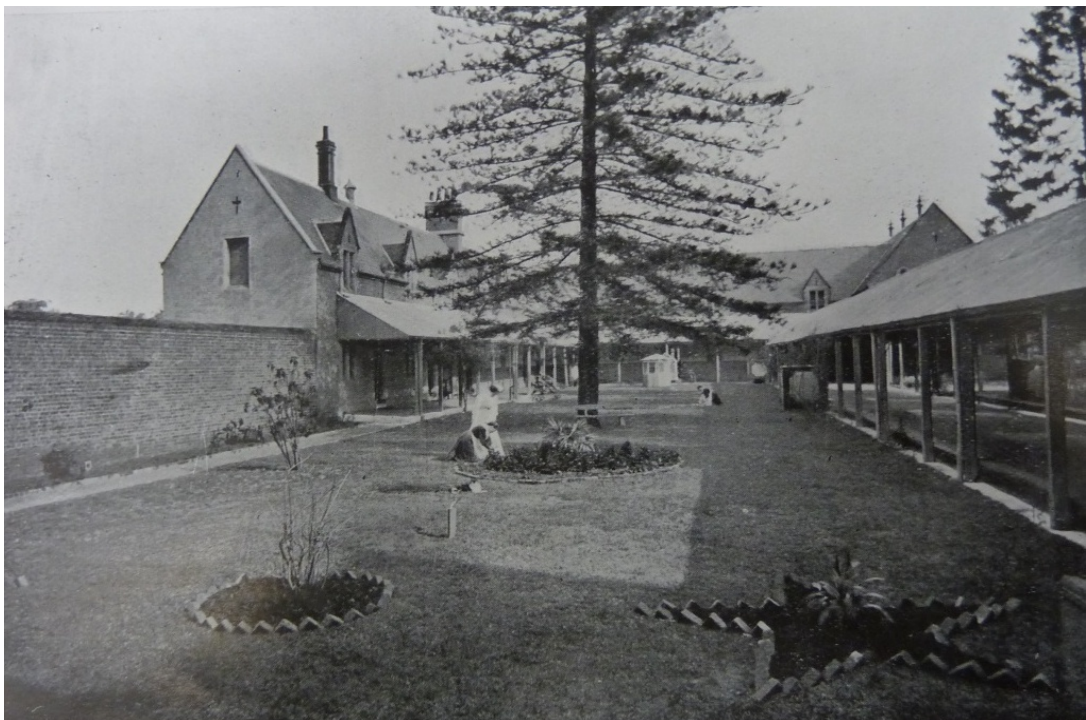
57 A c1910 view looking west in the courtyard of the Parramatta Industrial School for Girls, with the covered way at right leading to the Recreation Room (Chapel—c1858), Dining Room with Dormitory above (c1850) at centre and the Kitchen Annex with staff quarters above at left. This image shows that in the early twentieth century the landscape was well kept with brick edged circular and star-shaped beds popular at that time. Source: Parramatta Industrial School for Girls Annual Handbook, 1910.
