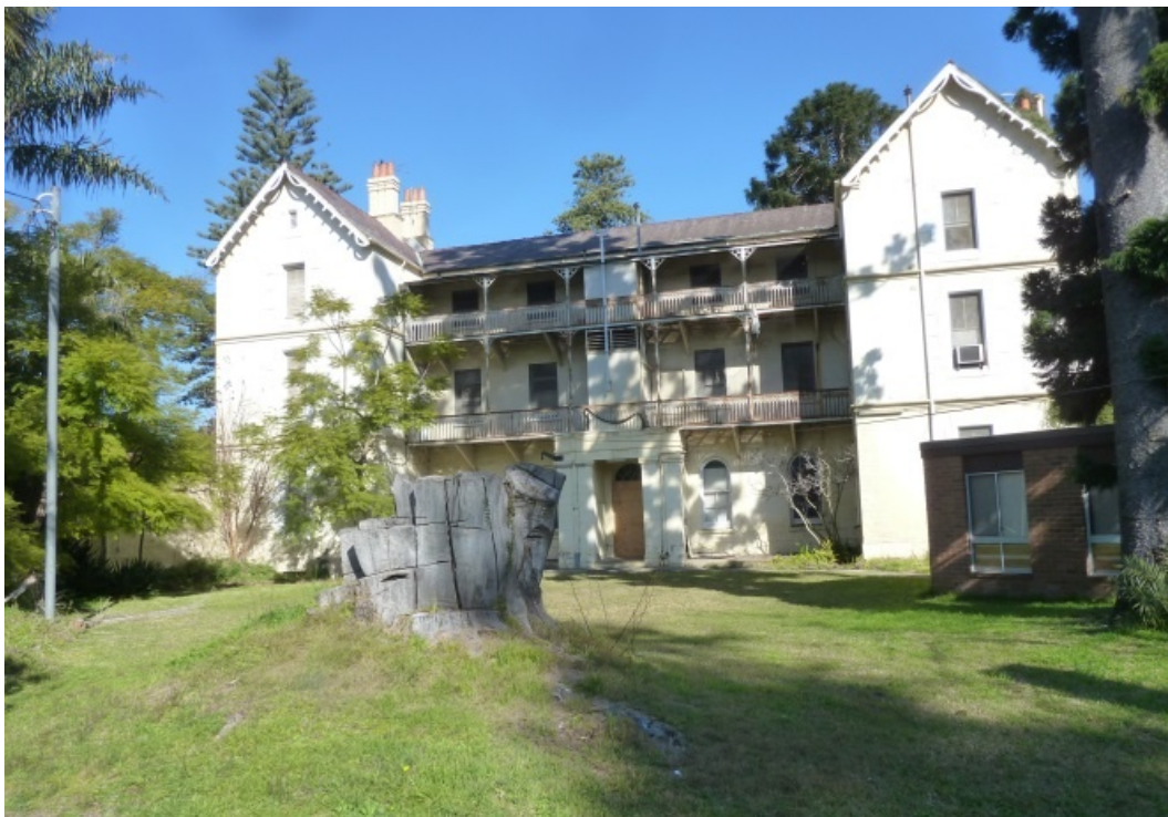
50 North-eastern elevation of Main Dormitory Block (Building N01), showing tall Araucarias at right and behind the building. Source: MUSEscape, October 2015.
