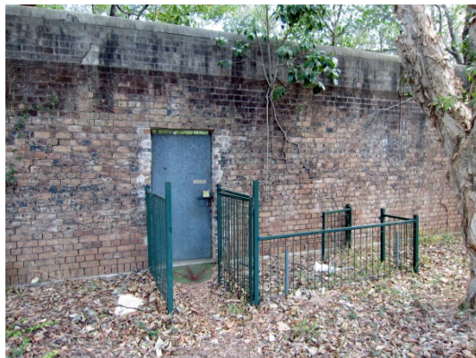
72 The brick perimeter wall. Note the later door opening and extension to the height of the wall. Source: TKD Architects, 2015.
