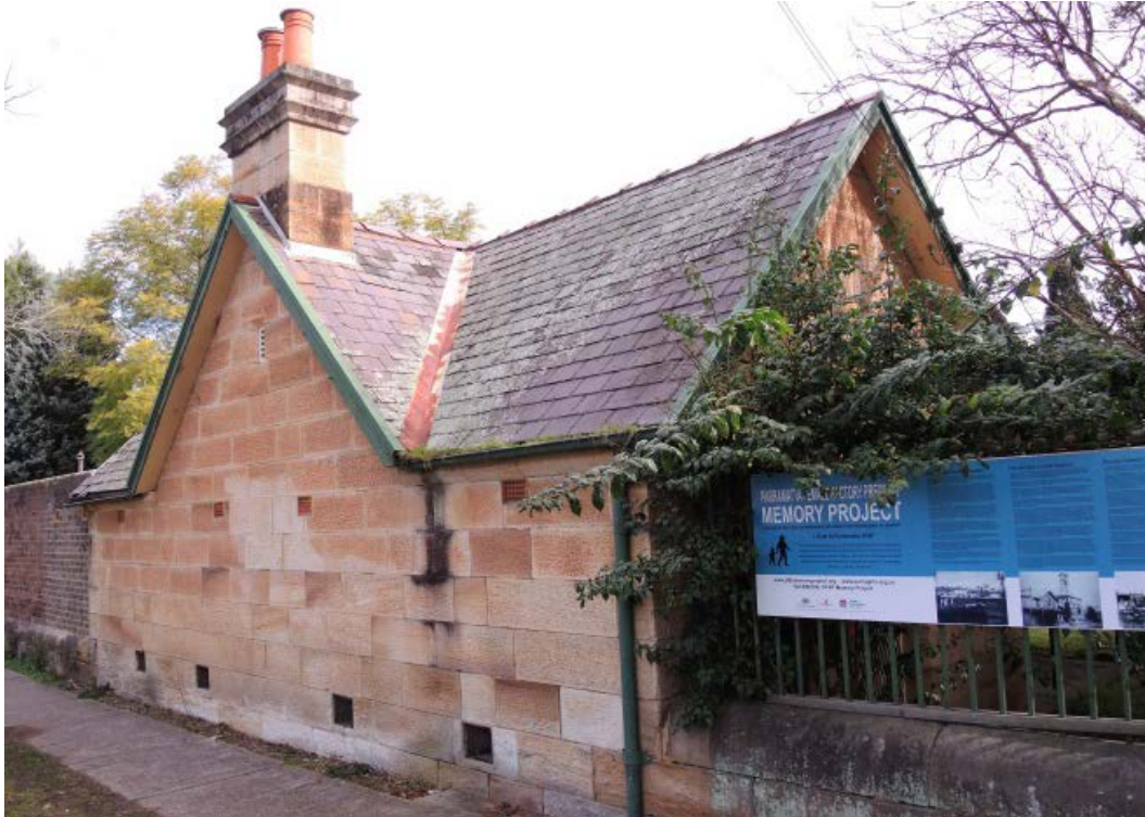
49 The Gatekeeper's Cottage (Building N07) next to the entrance to Norma Parker Centre / Kamballa from Fleet Street. The signs on the palisade fence tell the story of the Memory Project associated with the Parramatta Girls Home. Source: MUSEscape, October 2015.
