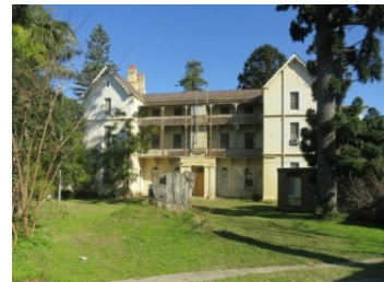
The c1844 Main Building (N01) of the Roman Catholic Orphan School with later additions—North Wing (1867) and South Wing (1882).
