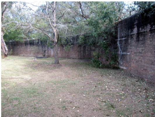
72 The brick perimeter wall. Note the later door opening and extension to the height of the wall. Source: TKD Architects, 2015.
